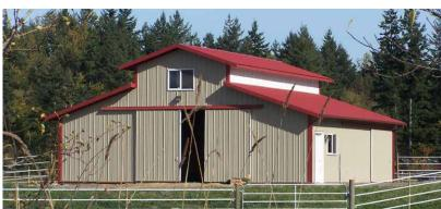
PBR Panel is ideal for pre-engineered metal, post-frame, and agricultural buildings. PBR Panel offers a unique yet flexible design when combined with other building materials is perfect for use in buildings for livestock and animal confinement.
